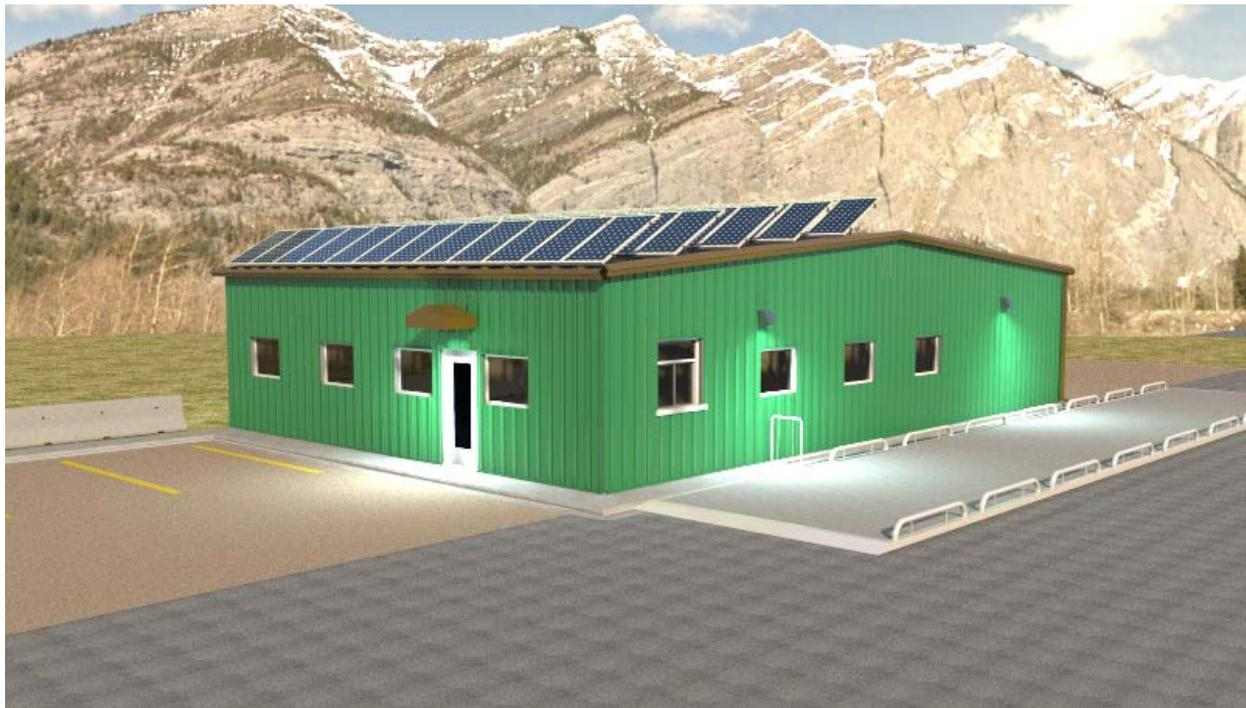
The solar panels are rated to -40c and the roof is designed to accommodate the panels and ensure the maximum exposure angle is achieved.
